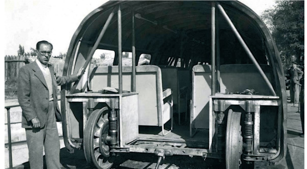
Rolling gear with independent free wheels in the Talgo I prototype
