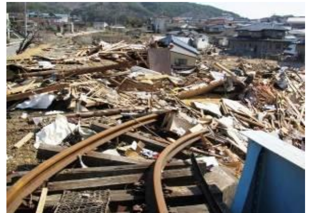
Tracks washed away by tsunami
