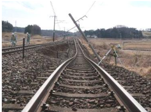
Collapsed embankment
