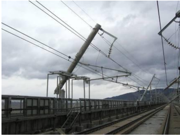
Toppled electrification masts
