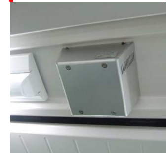
Beacon equipment (for Train Net)
